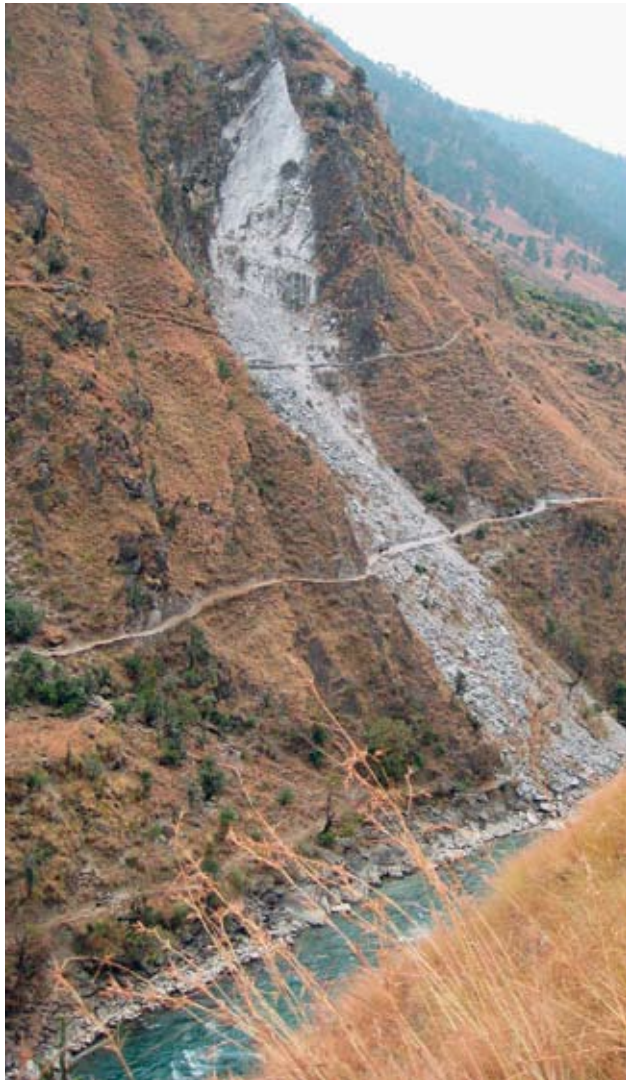
The two paths had to be cleared after the landslide before people could move from village to village again.
