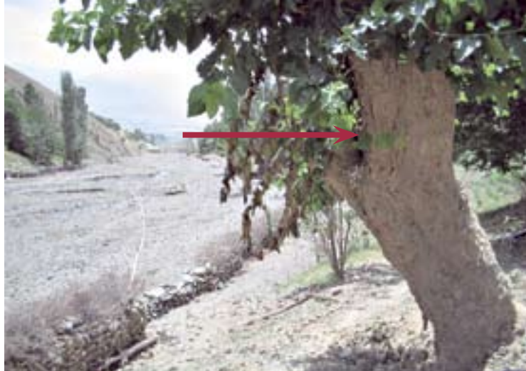
The arrow shows how high the mud reached that night in April. Down by the river you can see the small wall of stone that the desperate women build in fear of the next flood.
